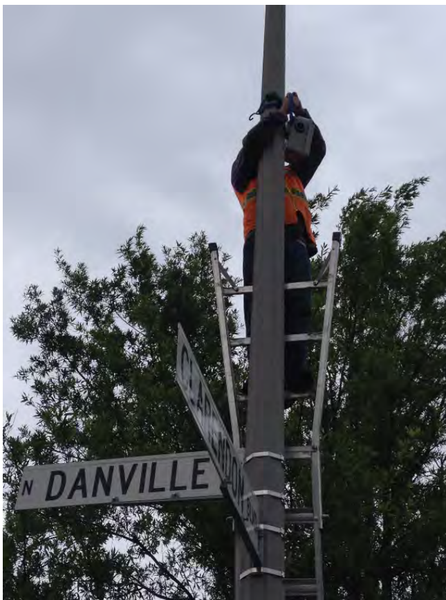
Figure A-9. Installing a Video Camera for Video Data Collection
